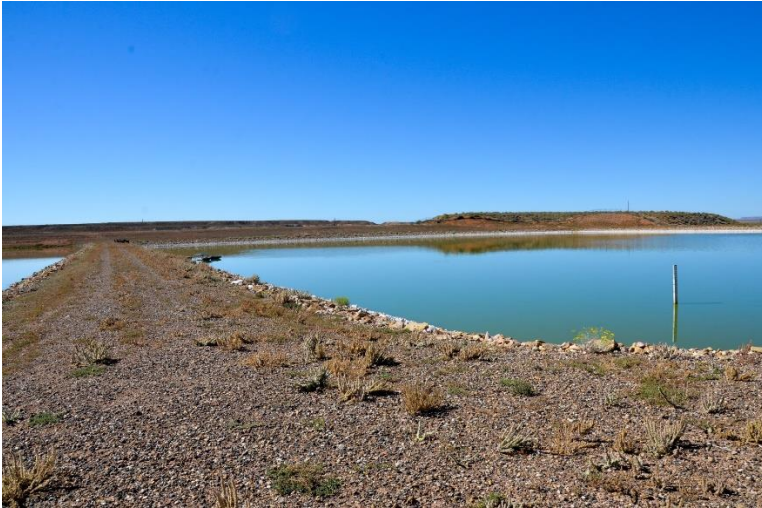
Figure 10: Wastewater Evaporation Pond
