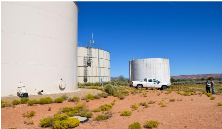
Figure 6: Fredonia Water Storage Tanks
