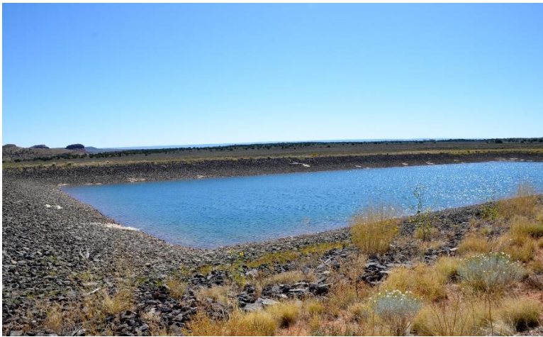
Figure 7: Fredonia Backwash Reservoir
